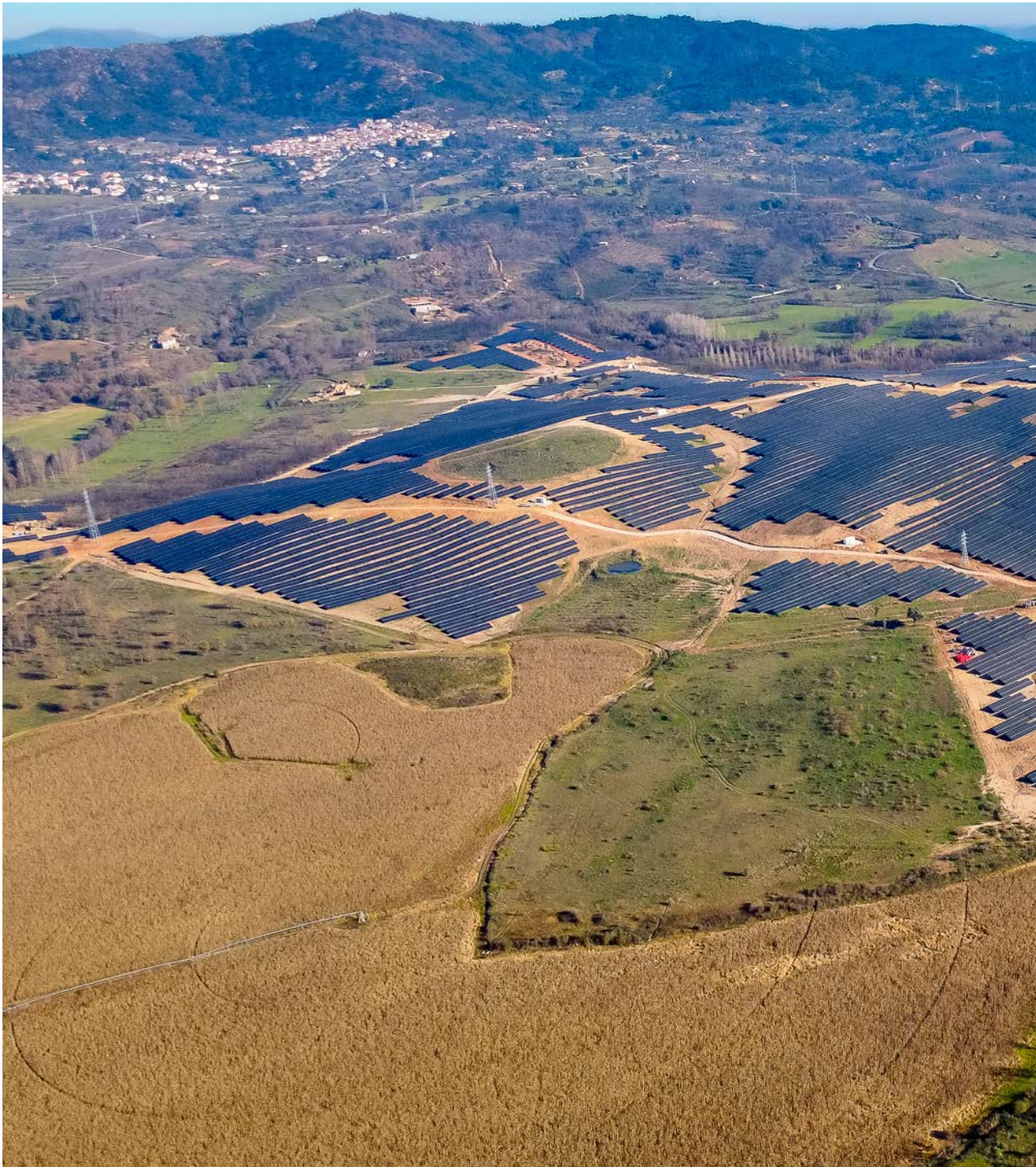
126.5 MW FUNDÃO PHOTOVOLTAIC PLANT + SUBSTATION 220 KV AND TRANSMISSION LINE (PORTUGAL)
