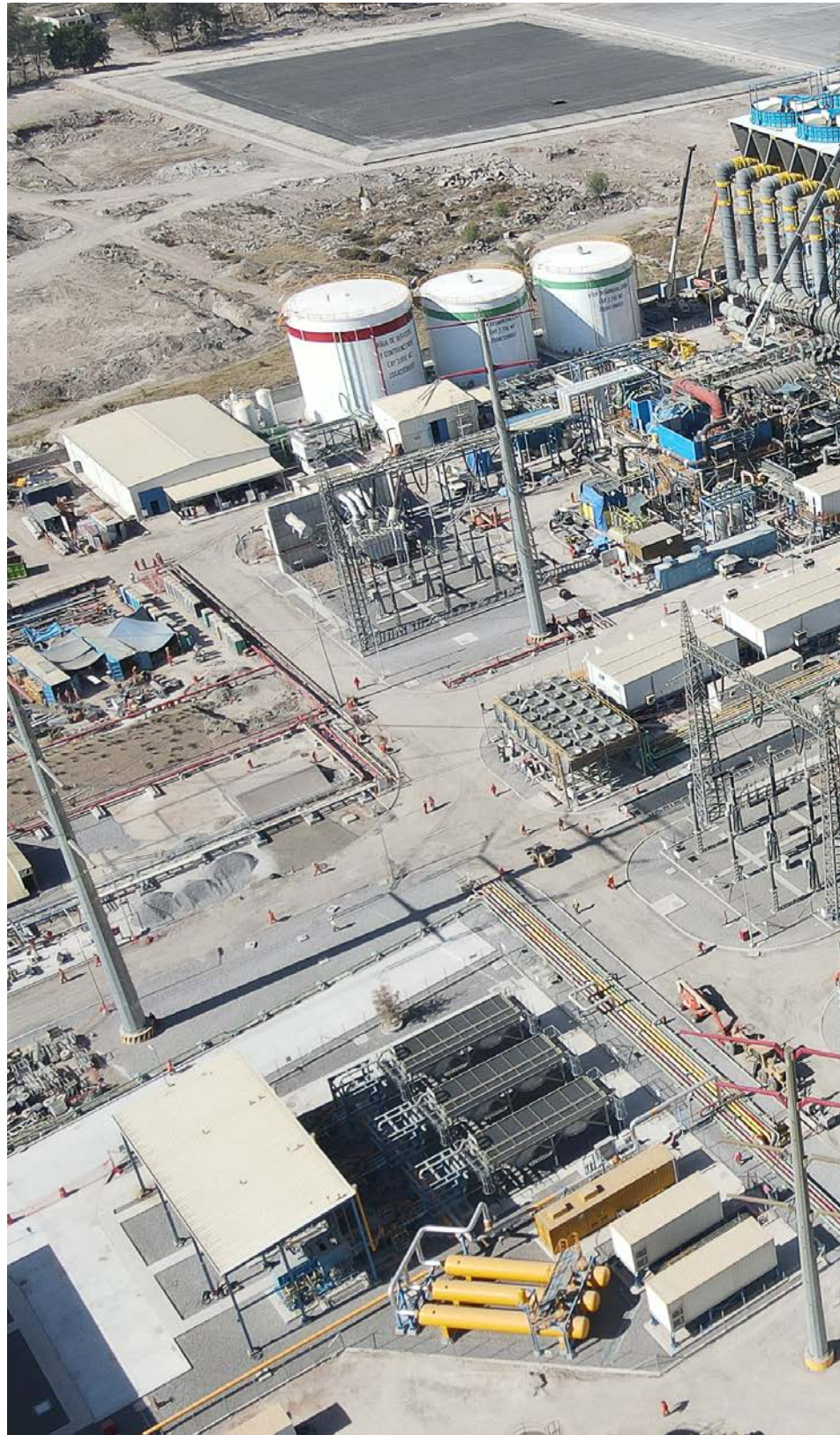
SALAMANCA 950 MW CCGT+ SUBSTATION 400 KV AND TRANSMISSION LINE (MEXICO)
