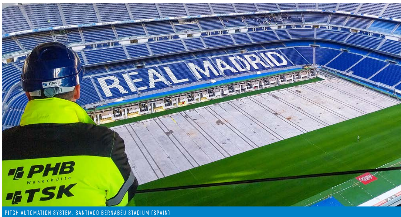
PITCH AUTOMATION SYSTEM. SANTIAGO BERNABÉU STADIUM (SPAIN)
