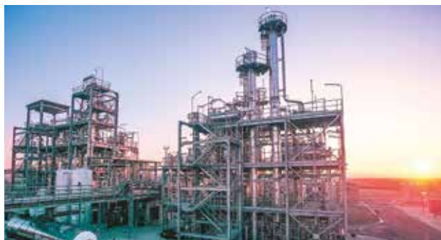
Caparrosa Biofuel Plant, Navarra (Spain)
