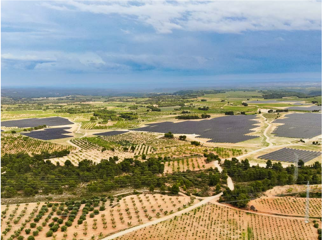
MINGLANILLA 100 MW SOLAR PARK + SUBSTATION + TL 132 KV (SPAIN)
