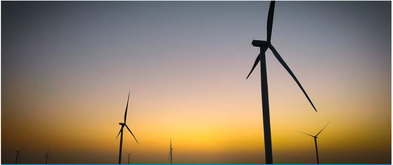
50 MW DHOFAR EOLIC PARK + 132 KV SUBSTATION (OMAN)
